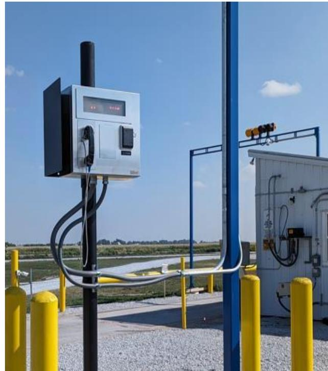
Once probing has completed, a buzzer will sound alerting truck to pull forward to the West inbound scale in front of them. There will be a space to stage until the truck in front finishes getting weighed in. Once on the scale, truck will pull up to the scale pedestal and swipe their card once more to initiate weighing of the truck.
